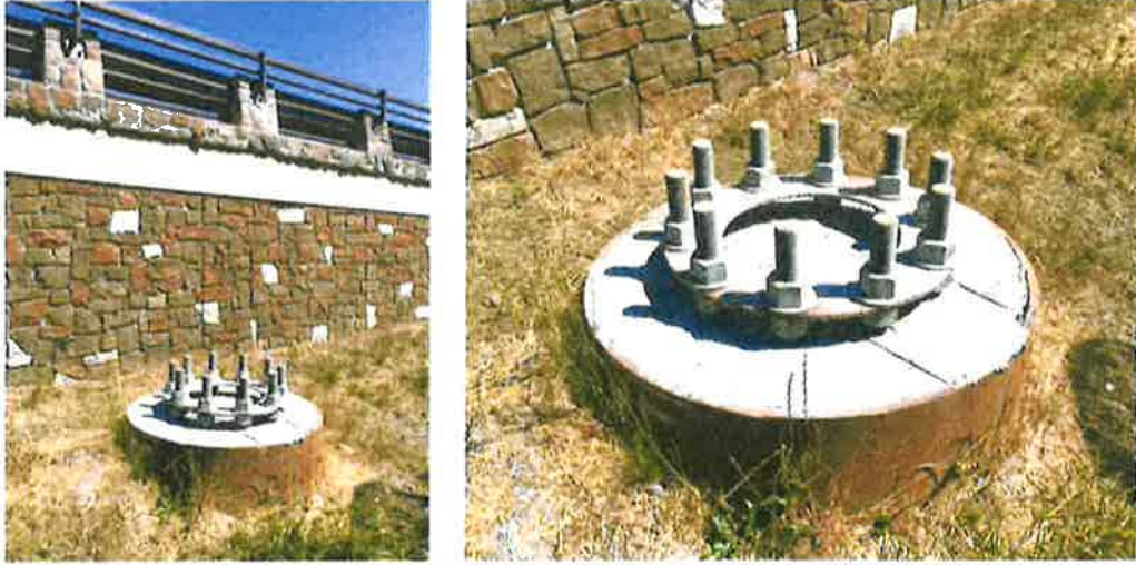
Existing Column Footings for Sebastopol Portals
